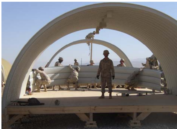
1st Platoon B/864th constructing K-huts in Sharana
