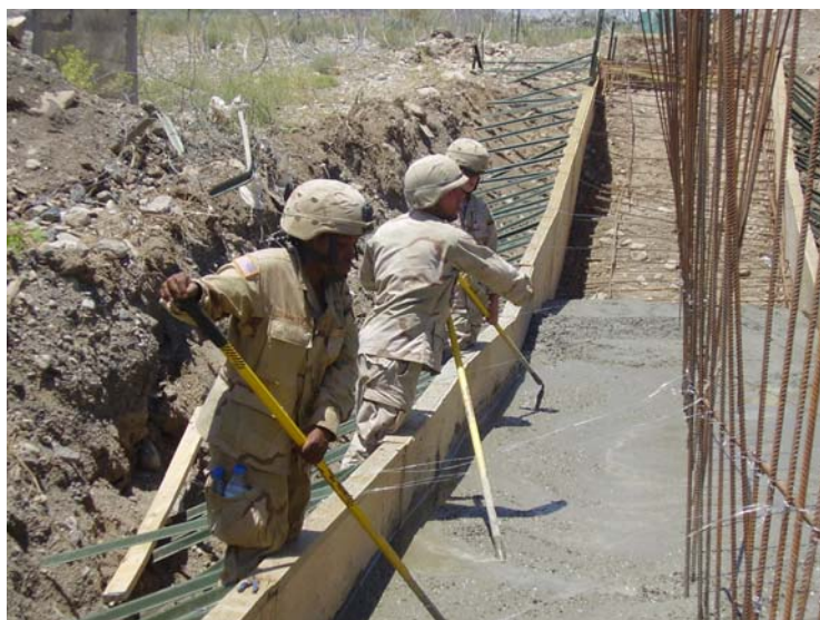
1st Platoon B/864th, placing concrete for North ECP in FOB Salerno.
