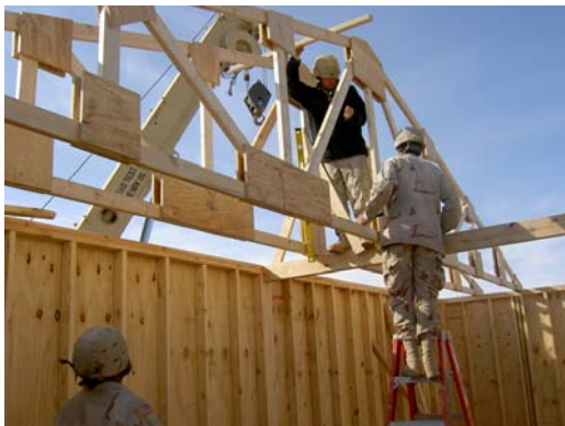
A/864th 1st Platoon, constructing Pole Barn 5.
