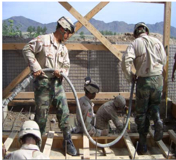
2nd Platoon B/864th, emplacing concrete for one of the five slabs.
